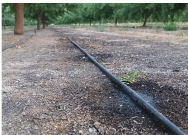
Figure 11. Drip irrigation system. (Photo by ANR Communications Advisory Board)
