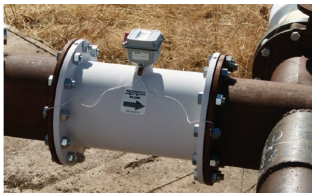
Figure 2. Electromagnetic flow meter, often referred to as a magmeter.
