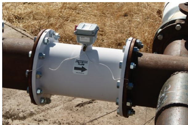
Figure 2. Electromagnetic flow meter, often referred to as a magmeter.
