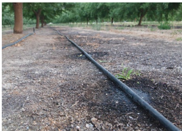
Figure 13. Drip irrigation system. (Photo by ANR Communications Advisory Board)
