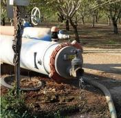
Leaks at filter .61 GPM 36.6 GPH 20,773 gal per irrigation season
